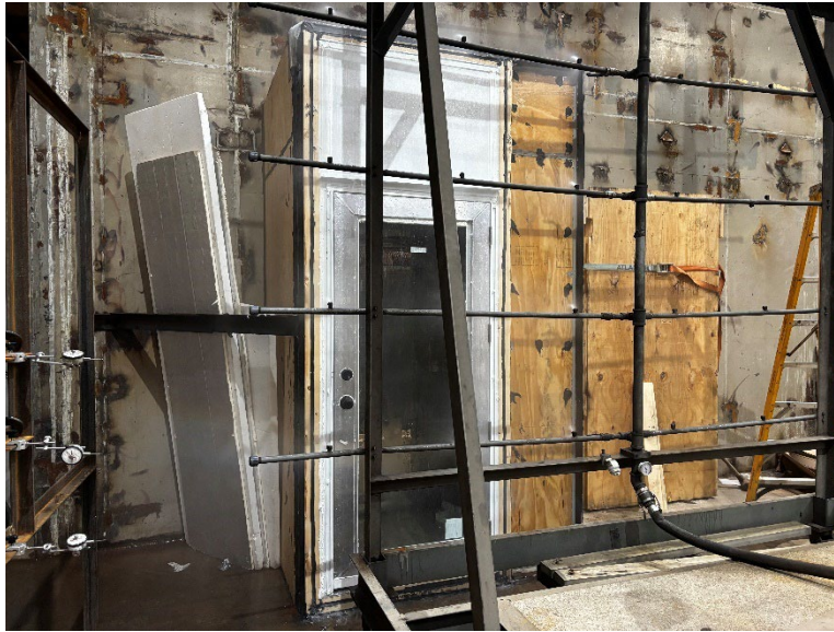
Photo No. 3 Static Water Penetration Testing
